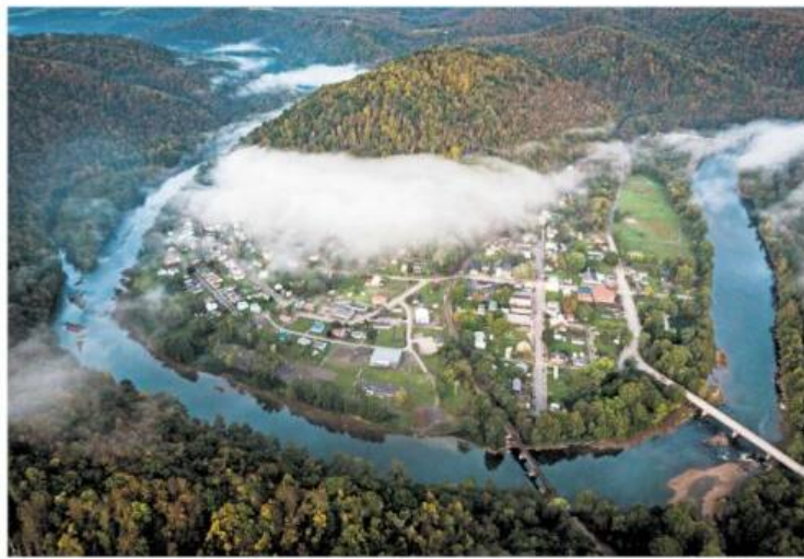
Rowlesburg's raw sewage spills into the Cheat River in heavy storms. Data finds no state more exposed to floods than West Virginia.
