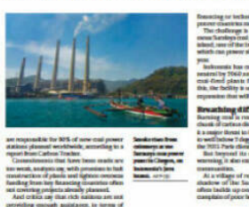
A large industrial facility, likely a coal power plant or processing plant, with tall smokestacks.
